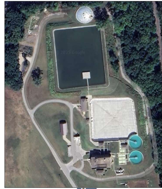
North Treatment Plant
