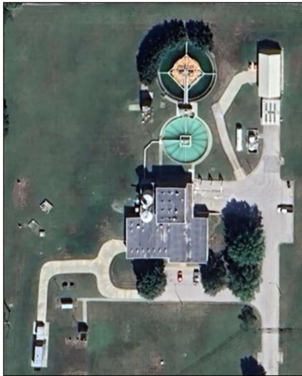
South Treatment Plant
